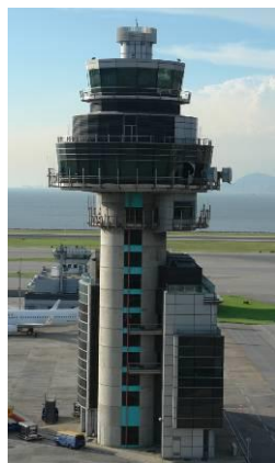
North Tower (N-TWR)
