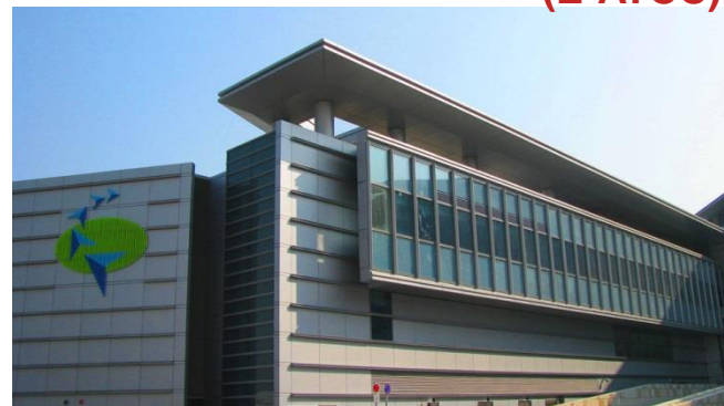
East ATC Centre (E-ATCC)
