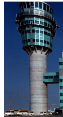
South Tower (S-TWR)
